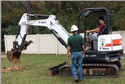
A Sheridan Construction superintendent helps students operate an excavator at the Macon event.
