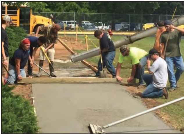
R. W. Allen, LLC taught students at Evans High School how to pour concrete for a sidewalk. Both the principal and instructor were appreciative of this involvement and said the students were eager for the next opportunity.
