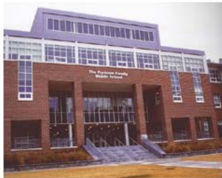
Tebarco Mechanical Corporation Lovett New Middle School Atlanta
