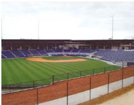
Precision Concrete Construction, Inc. Gwinnett Braves Stadium Lawrenceville
