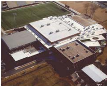
Tebarco Mechanical Corporation Woodward Academy Athletic Complex College Park
