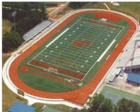
Sports Turf Company, Inc. North Springs High School Stadium Field & Track Renovation Sandy Springs
