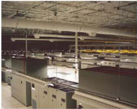
Eckardt Electric Company AT&T Lithia Springs Internet Data Center Expansion Lithia Springs
