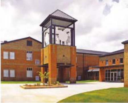
Parrish Construction Group Howard High School Macon
