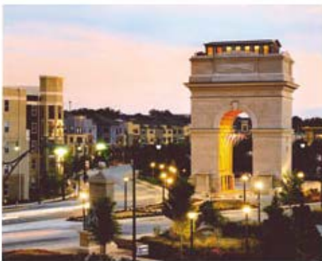
New South Construction Co., Inc. The Millennium Gate Atlanta
