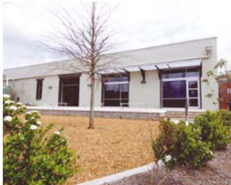
Gay Construction Company Trees Atlanta Headquarters Atlanta Also took First Place in the Best Sustainable Building Practices Division
