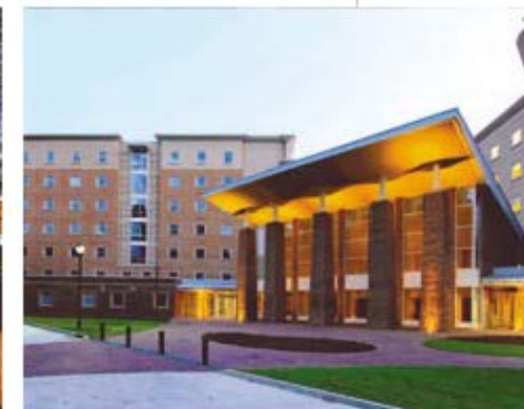
New South Construction Co., Inc. Spelman College - Student Housing, Dining and Parking Deck Atlanta
