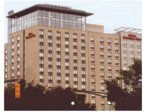
Holder Construction Company Aquarium Hilton Garden Inn Atlanta
