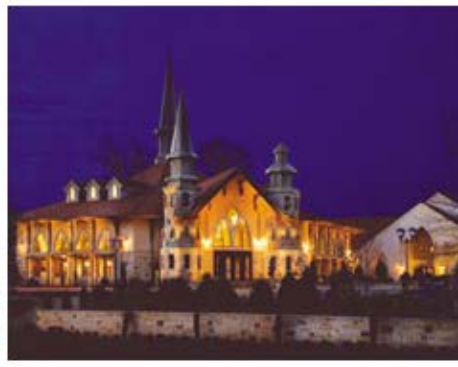
Cork-Howard Construction Catholic Church of St. Ann, Narthex & Nave Renovation Marietta
