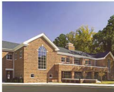
New South Construction Co., Inc. Peachtree Presbyterian Church Campus Addition & Renovation Atlanta
