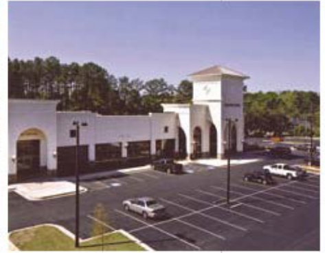
Hogan Construction Group, LLC. Butts County Administration Building, Superior Court Clerk's Offices & Library Renovation Jackson
