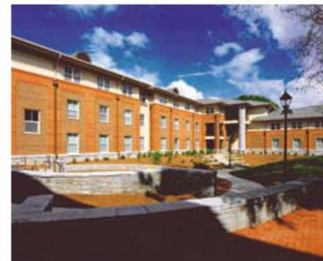
New South Construction Co., Inc. Oxford College of Emory University New Residence Hall Complex Oxford
