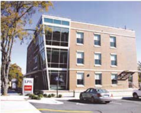
Saliba Construction Company Lindsay Professional Office Building Lawrenceville
