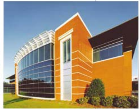
International City Builders, Inc. Flint Energies Member Service Center Warner Robins
