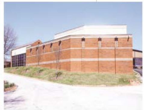
Carroll Daniel Construction Co. Lakeview Academy CAmpus Expansion Phase 1 Gainesville
