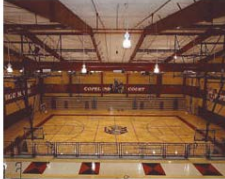
Piedmont Construction Group, LLC Northeast High School Macon
