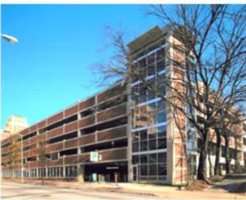
C. D. Moody Construction Company Downtown Parking Deck Atlanta, GA
