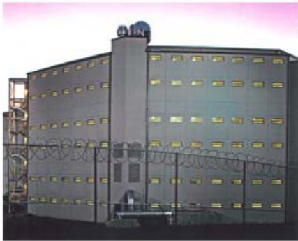
Turner Construction Company Hall County Jail and Core Support Center Gainesville, GA
