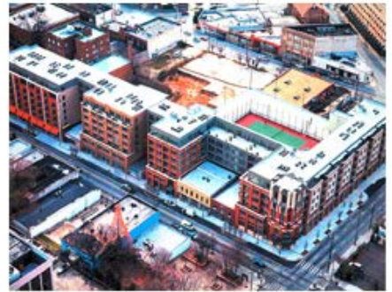
J.M. Wilkerson Construction Co., Inc. Renaissance Walk at Sweet Auburn Atlanta, GA
