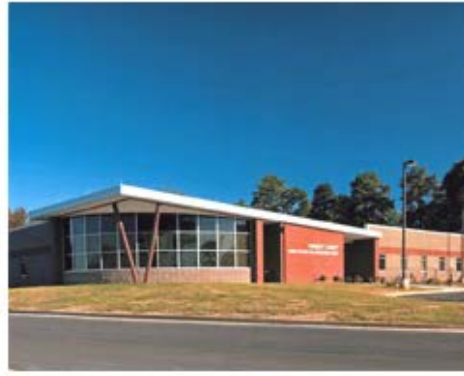
Rogers Construction Company Gwinnett County Animal Welfare and Enforcement Center Lawrenceville, GA
