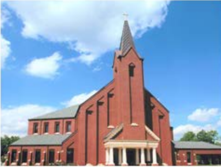
Carroll Daniel Construction Company St. John Baptist Church Gainesville, Georgia
