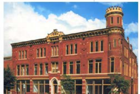
Garbutt Construction Company Restoration and Renovation of the Macon Volunteers Army Macon, Georgia
