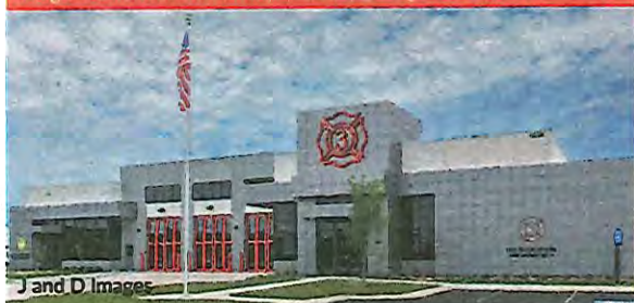
Forest Park Gillem Public Safety Building | Hogan Construction Group | New | Design-Bid-Build
