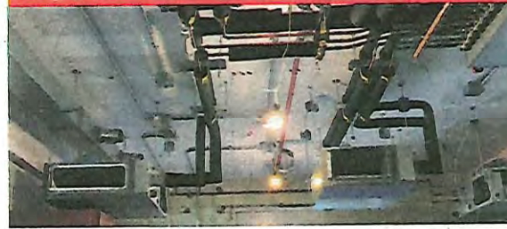
The University of Georgia, Hoke Smith Annex HVAC Upgrades | Piedmont Construction Group | Renovation | Design/Build
