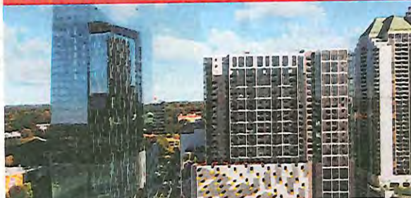
Midtown Union | Brasfield & Gorrie | New | Construction Management at Risk
