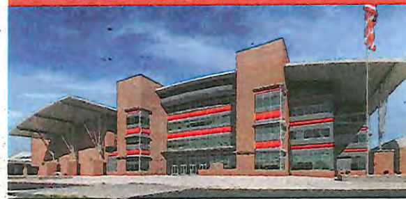
Lowndes High School | JCI Contractors | New | Construction Management at Risk
