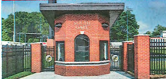
Calhoun High School Athletics Addition | SmithBuilt Construction Group | New | Design-Bid-Build
