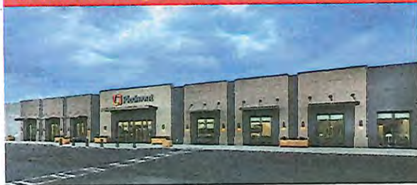
Piedmont Physician's Group Newton - Martin's Crossing | McCarthy Building Companies, Inc. | Renovation | Construction Management at Risk
