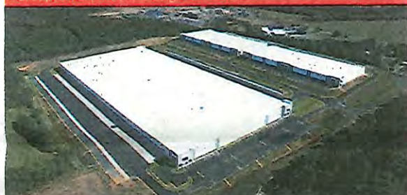
Cass White Logistics Center | Kajima Building & Design Group, INC. | New | Design-Bid-Build
