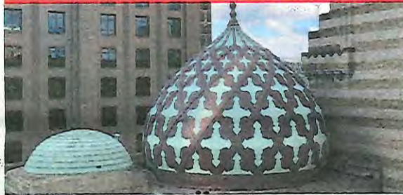
The Fox Theatre Onion Dome Renovation | Gay Construction Company | Renovation | Design-Bid-Build
