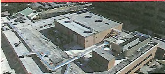
Phoebe Putney Memorial Hospital O.R. Penthouse Addition &amp; Renovation | Pellicano Construction | Renovation | Construction Management at Risk
