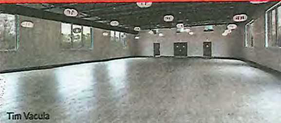
Emery Thomas Auditorium Renovation | Garbutt Construction Company | Renovation | Construction Management at Risk
