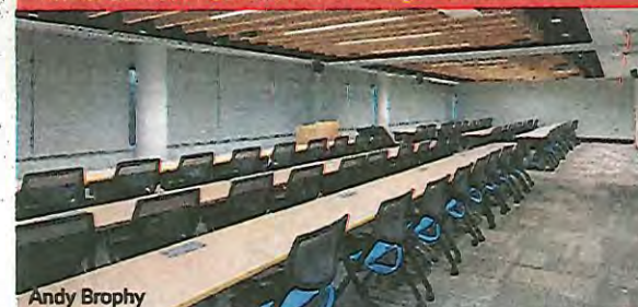
The Task Force for Global Health | Leapley Construction | Interior Buildout | Construction Management at Risk
