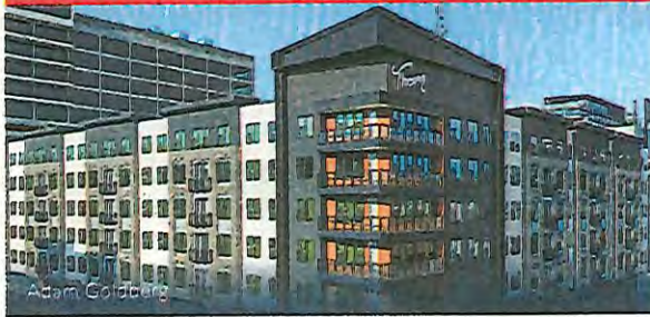
Interlock Phase II (Mixed-Use) | Choate Construction New | Construction Management at Risk
