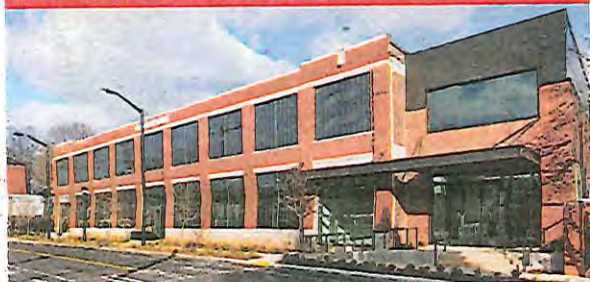
560 Edgewood | Balfour Beatty | Renovation | Construction Management at Risk
