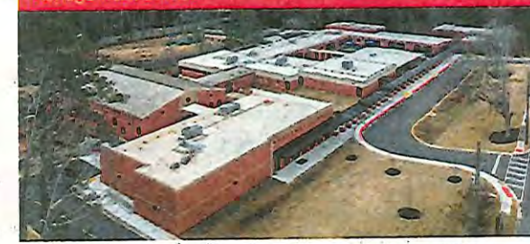
West Side Elementary School Renovation and Addition Parrish Construction Group | Renovation | Construction Management at Risk
