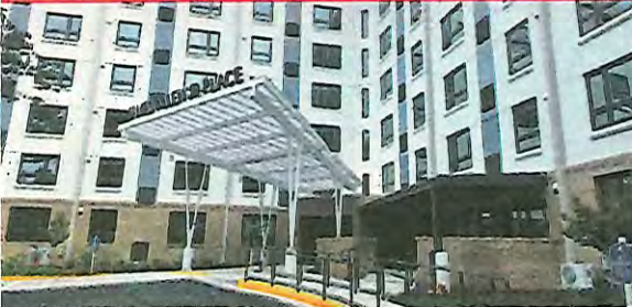
Hightower Manor | J.M. Wilkerson Construction Co., Inc. | Renovation | Design-Bid-Build
