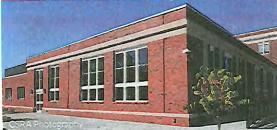
Savannah Arts Academy Addition and Renovation | McKnight Construction | Renovation | Construction Management
