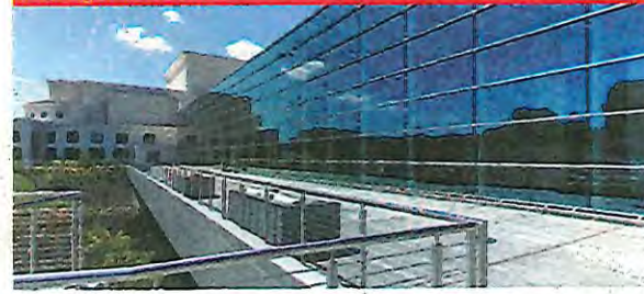
Gas South District Renovation and Expansion Holder Construction Company | Renovation | Construction Management at Risk
