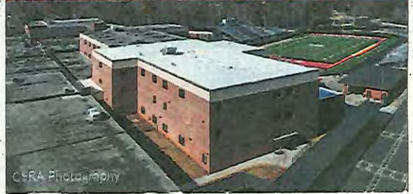
North Gwinnett High School East Wing Addition | McKnight Construction | New | Design-Bid-Build
