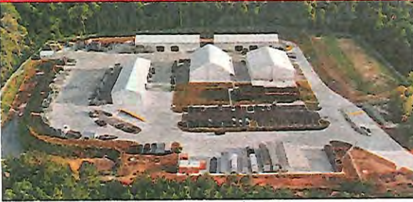
Flex TC - Villa Rica Development | Caliber 1 Construction | New | Design-Bid-Build
