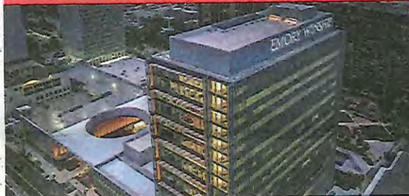
Winship Cancer Institute at Emory Midtown | Batson-Cook Construction | New | Construction Management at Risk
