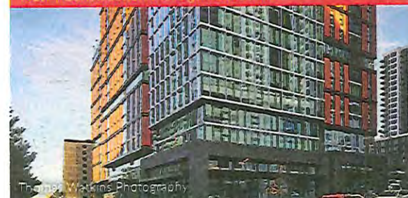
Hub Atlanta | Juneau Construction Co. New | Construction Management at Risk
