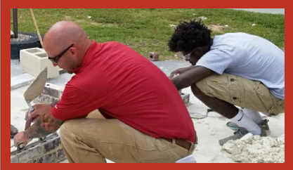
Elkins Construction helped students at Statesboro High School with masonry skills.
