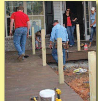
Responding to the Halstead family's need to ready their home in Jefferson to accommodate their child with severe brain damage, YLP members stepped in and built a wheelchair-accessible deck and front entrance ramp.
