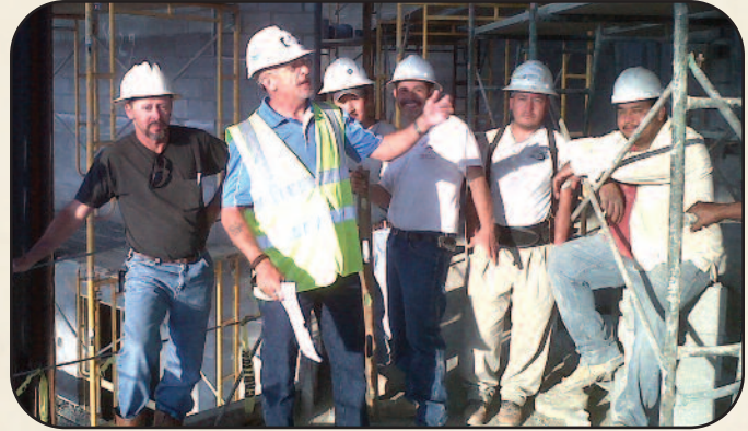
Participating in the recent Safety Stand Down focusing on scaffold training helps to insure a safer workforce.
