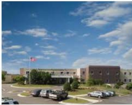
Rawlins Mechanical Contractors, Inc. Piedmont Mountainside ED and Surgery Addition Jasper
