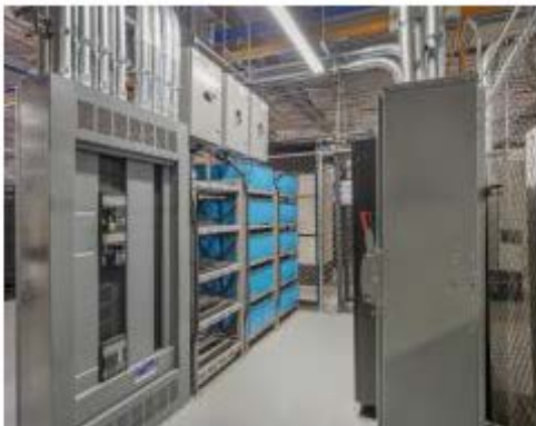
Eckardt Electric GNAX Fourth Electrical Service Atlanta
