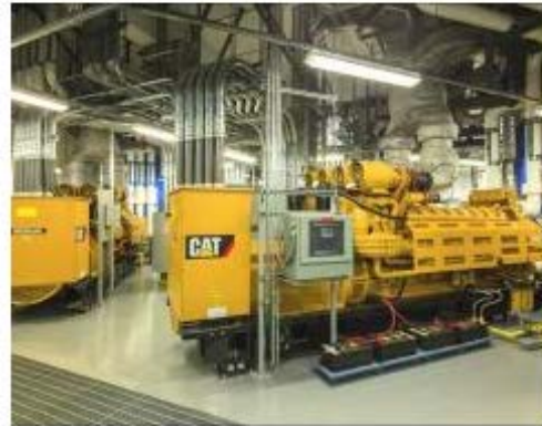
Eckardt Electric 51 Peachtree Center Avenue Generator and UPS Replacements Atlanta
