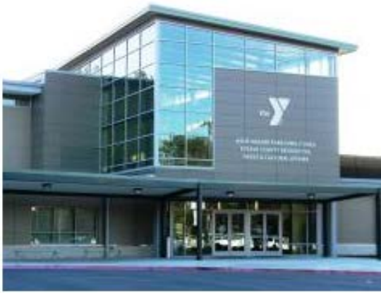
Taylor Commercial, Inc. Wade Walker Park Multi-Purpose Aquatic Center Stone Mountain
