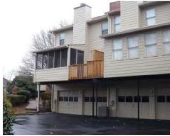
Taylor Commercial, Inc. Windsor Trace Condominiums Norcross
