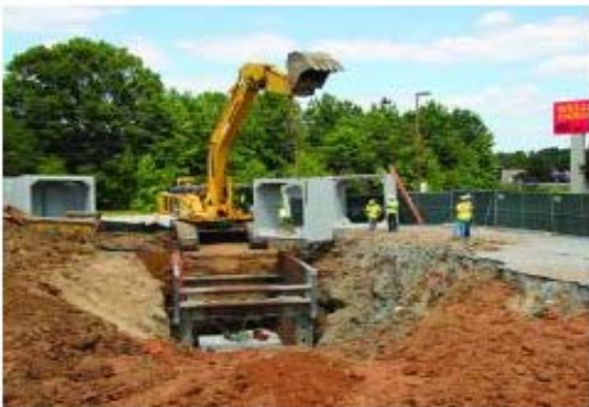
Brent Scarbrough & Company, Inc. Wells Fargo Emergency Storm Culvert Repair Columbus
