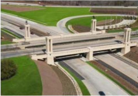
Athena Construction Group The New Gateway to Fort Benning Columbus
