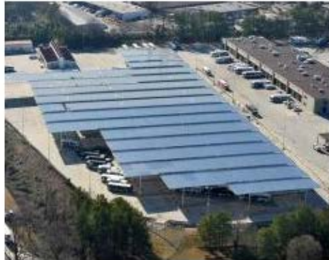
LeMay Electric, Inc. MARTASUN Solar Canopy at the Laredo Drive Bus Maintenance Facility Decatur
