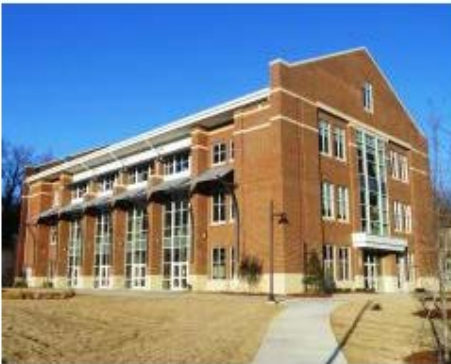
Tebarco Mechanical Corporation Atlanta International School New Art, Science & Design Center Atlanta
