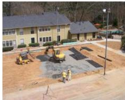
Brent Scarbrough & Company Rockledge Apartments Marietta
