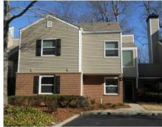
Taylor Commercial, Inc. The Arbor Condominiums Atlanta
