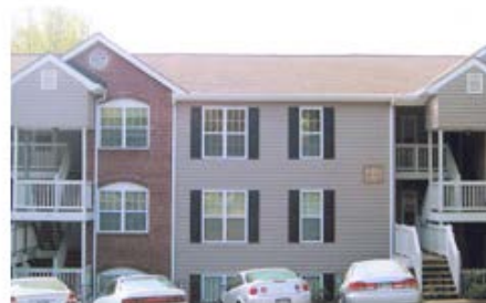
First Place Taylor Commercial, Inc. Martin Lakes Condominiums Roswell, Georgia
