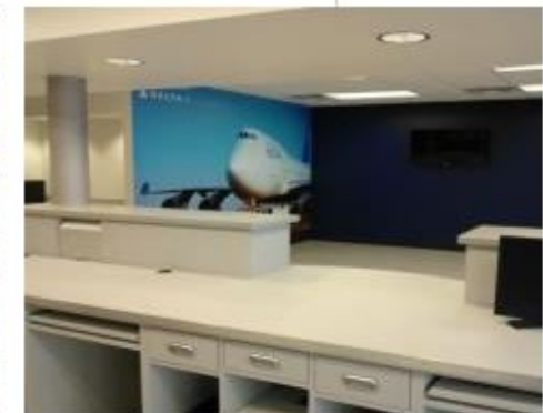
Green Heart Enterprises Delta Airlines Cargo Breezeway Renovation Atlanta
