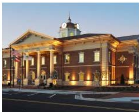
Van Winkle Construction Sugar Hill City Hall Sugar Hill
