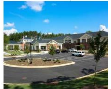
Piedmont Construction Group Ansley Park Health and Rehabilitation Newnan
