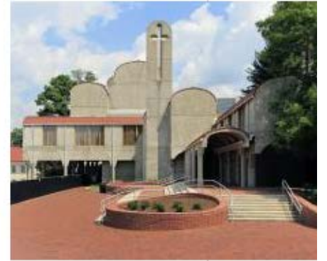
New South Construction Company Emory University - Cannon Chapel Technology Interior Renovation Project Atlanta
