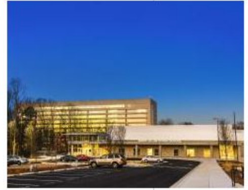
JE Dunn Construction Company Atlanta Public Schools New North Atlanta High School Atlanta
