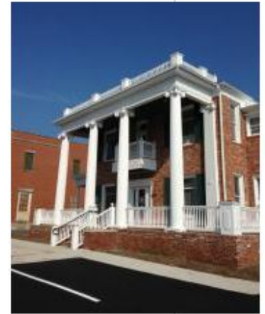
Garbutt Construction Company Community Bank of Dublin-Laurens County Restorations to 605 Bellevue Ave Dublin
