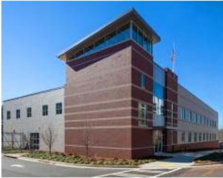
Hogan Construction Group, LLC Decatur Public Works Facility Decatur
