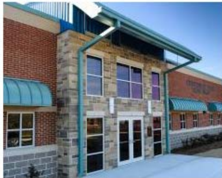
Parrish Construction Group Centerville Law Enforcement Center & Municipal Court Centerville
