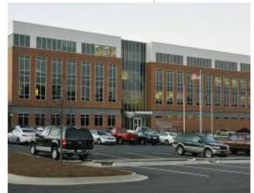
Turner / New South Joint Venture Douglas County Adult Detention & Law Enforcement Center Douglasville Also earned First Place in Best Sustainable Building Practices Division
