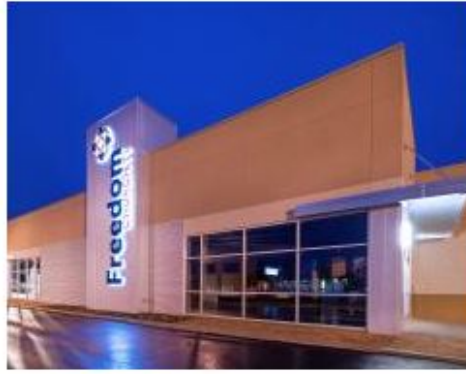
Hogan Construction Group, LLC Freedom Church Renovation Acworth
