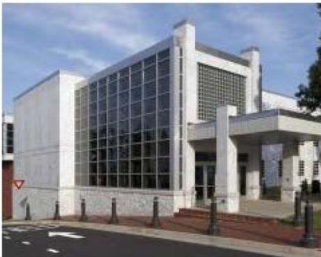
New South Construction Company Pickens County Courthouse Renovation and Expansion Jasper
