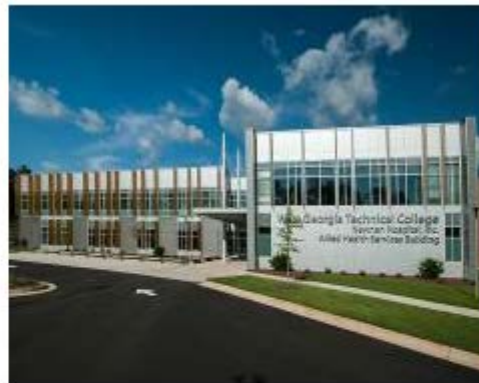
R. K. Redding Construction, Inc. Allied Healthcare Building Newnan
