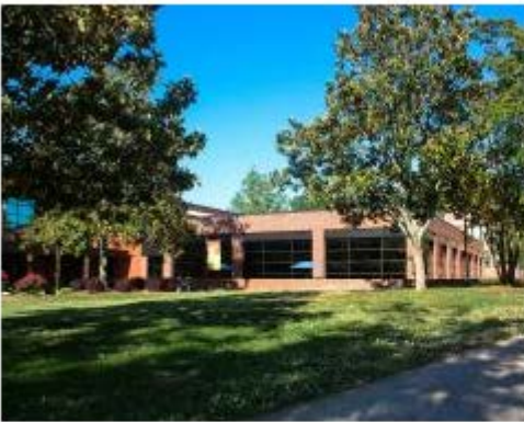
Piedmont Construction Group Gordon State College Dining Hall Renovations and Additions Barnesville
