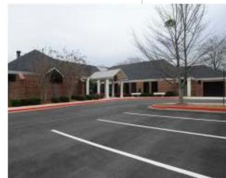
Hogan Construction Group, LLC Powder Springs Municipal Court Renovation Powder Springs
