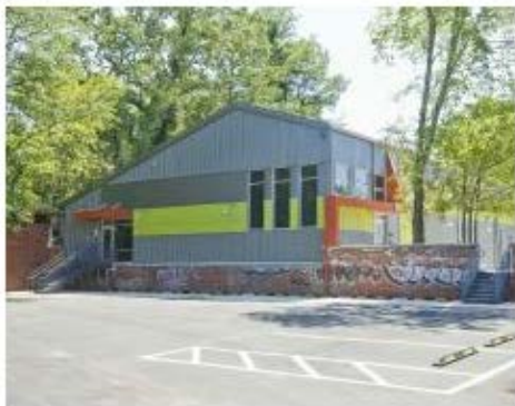
Derucki Construction Company Big Nerd Ranch Atlanta
