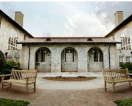
Holder Construction Company Emory University Dobbs Hall Renovation Atlanta Also earned First Place in Best Sustainable Building Practices Division
