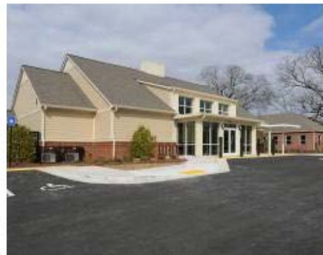
Hogan Construction Group / Bryson Constructors Joint Venture Oak Hill Child, Adolescent and Family Center Atlanta
