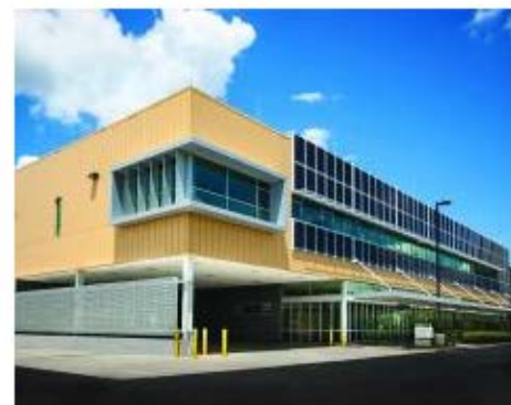
Gilbane Building Company Carbon Neutral Energy Solutions Lab Georgia Tech Atlanta Also earned First Place in Best Sustainable Building Practices Division
