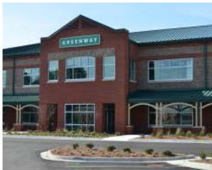
RA-LIN and Associates, Inc. Greenway Medical Technologies Corporate Headquarters Expansion Carrollton Also earned Merit Honors in the Best Sustainable Building Practices Division
