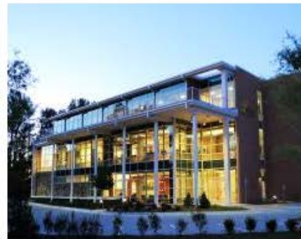
Choate Construction Company Palmetto Health Council Medical Office Building Palmetto Also earned First Place in Best Sustainable Building Practices Division
