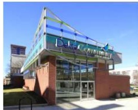
New South Construction Company Delta Community Credit Union - Midtown Atlanta
