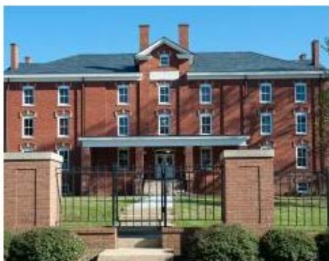
Garbutt Construction Company The Rehabilitation of Huntington Hall Fort Valley
