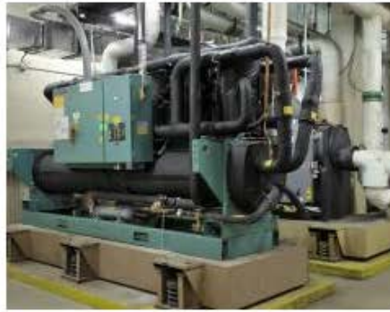
Parrish Construction Group HVAC Renovation - Atlanta Technical College Atlanta
