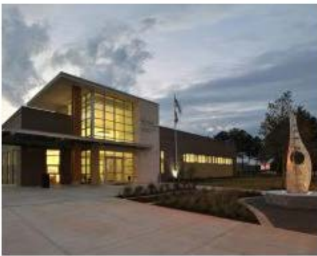
Hogan Construction Group, LLC Suwanee Police Substation and Training Suwanee
