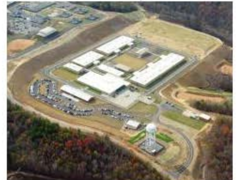
New South Construction Company Riverbend Correctional Facility Milledgeville
