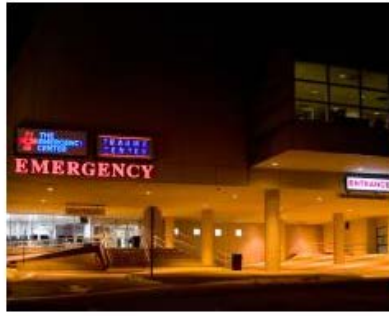
Warren Associates, Inc. Emergency Center Renovations - Medical Center of Central Georgia Macon
