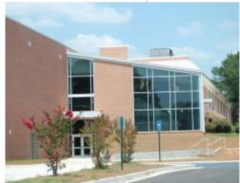
Hogan Construction Group, LLC Clarkston High School Renovation & Addition Clarkston
