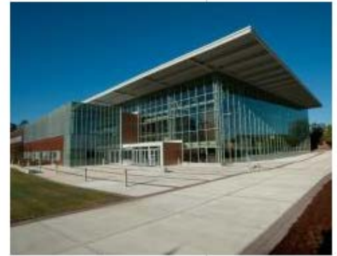
Garbutt/Christman Joint Venture Partnership The Wellness & Recreation Center at Georgia College and State University Milledgeville
