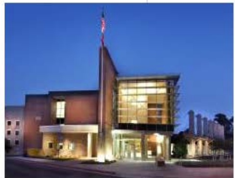
JE Dunn Construction Company Atlanta Public School System North Atlanta High School Remodel Atlanta
