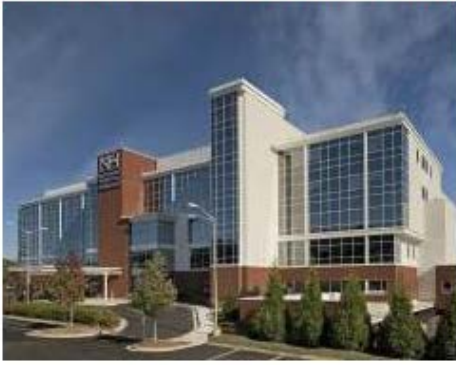
Batson-Cook Company Northside Hospital Forsyth Vertical Addition - West Cumming
