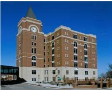
Turner Construction Company Cobb County Superior Court Marietta Also earned First Place in Best Sustainable Building Practices Division
