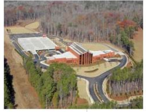
Cooper & Company General Contractors, Inc. Zion Hill Baptist Church, Phase 1 - Sitework, Parking Deck and Worship Center Atlanta
