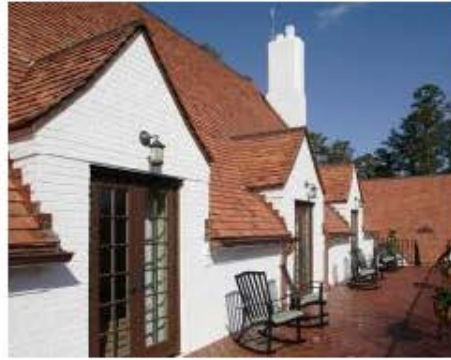
Gay Construction Company Normandy Inn at WinShape Retreat Mt. Berry
