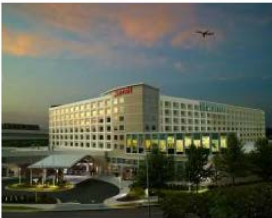
Brasfield & Gorrie Atlanta Airport Marriott Gateway College Park
