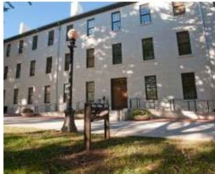
Garbutt Construction Company Renovation of New College Athens
