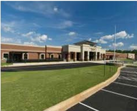
R. K. Redding Construction, Inc. Paulding County High School Addition Dallas Also took a Merit Award in the Best Sustainable Building Practices Division
