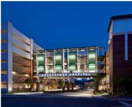
Brasfield & Gorrie WellStar Kennestone Hospital Cancer Center Deck Vertical Expansion Marietta
