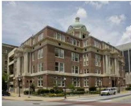
Chris R. Sheridan & Company Renovations to Bibb County Courthouse Macon
