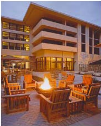
Turner Construction Company Emory Conference Center Hotel Expansion & Renovation Atlanta Also took a Merit Award in the Best Sustainable Building Practices Division
