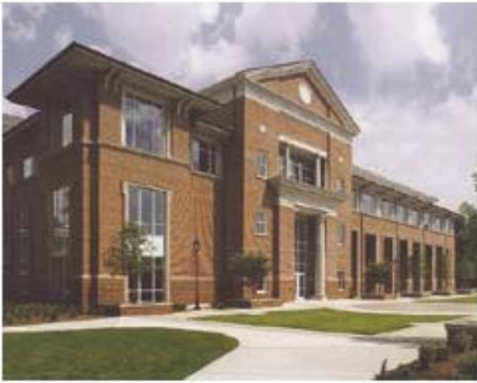
Holder Construction Company Tate Student Center Expansion at the University of Georgia Athens
