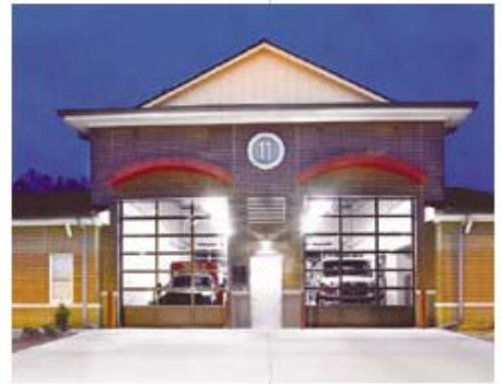
Hogan Construction Group, LLC Paulding County Fire Station 11 Acworth
