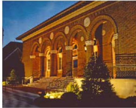
S.C. Barker Construction Tifton-Tift County Public Library Tifton Also took a Merit Award in the Best Sustainable Building Practices Division
