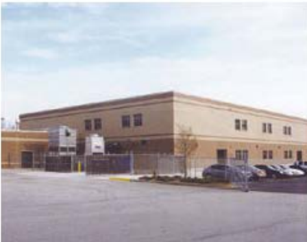
Carroll Daniel Construction Company Addition and Alterations to Chesney Elementary School Duluth
