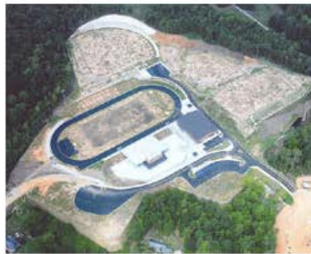
Swofford Construction, Inc. Lanier High School Athletics Facilities Sugarhill
