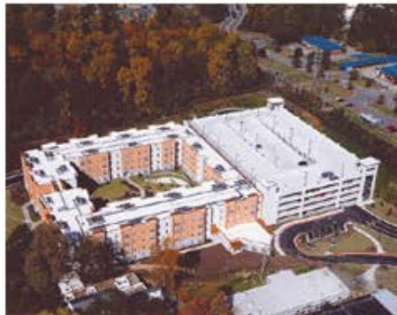
Young Contracting/SE, Inc. Life University Residence Hall/Parking Deck Marietta Also took First Place in the Best Sustainable Building Practices Division
