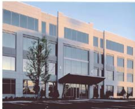
Choate Construction Company - Atlanta Federal Aviation Administration Headquarters Hapeville
