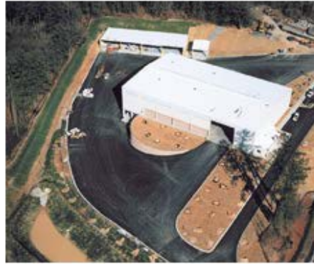
Lusk & Associates, Inc. Plant Atkinson MSW Transfer Station Smyrna, Georgia
