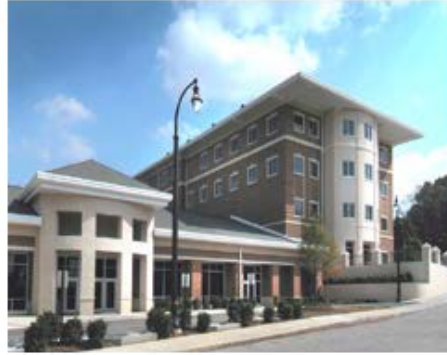
C.D. Moody Construction Company, Inc. The Leadership Center at Morehouse College Atlanta, Georgia
