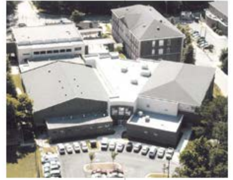
New South Construction Company, Inc. Atlanta International School- Sports & Activities Center Atlanta, Georgia
