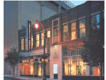
Gay Construction Company The Balzer Theater at Herren's Atlanta, Georgia
